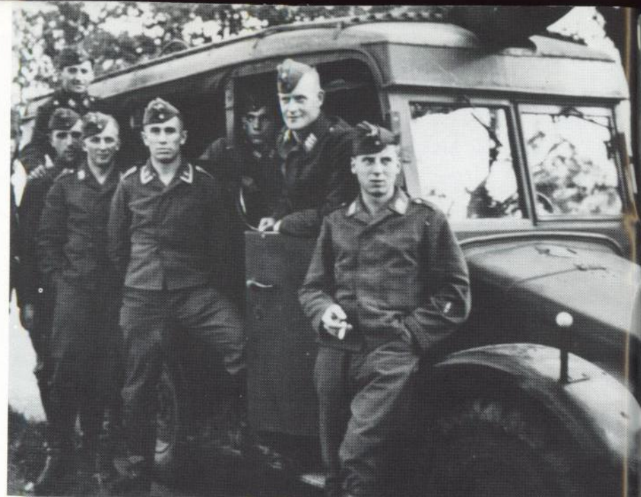
Above: Krupp L 2 H 143 as telephone truck (Kfz.19). Crew: driver and five men. It is not known why this vehicle was not introduced as Kfz.61.
